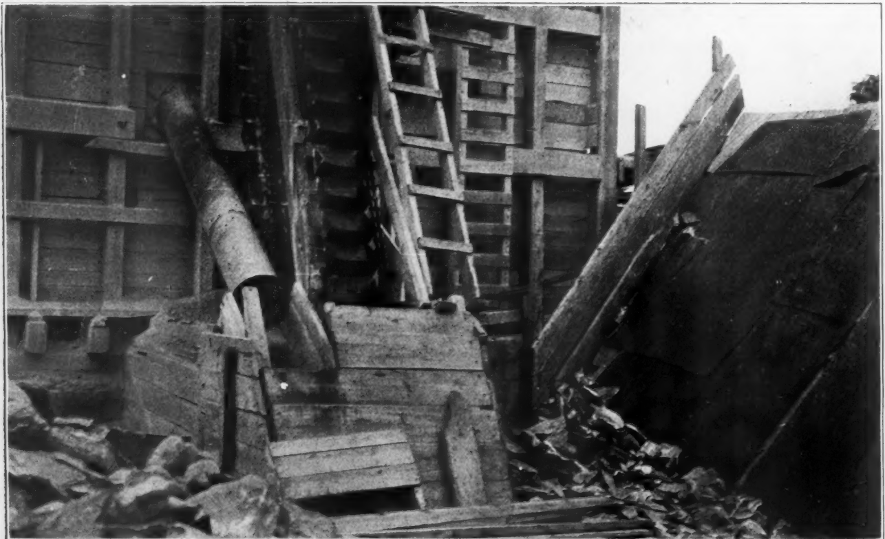
Chute Down Which Quarry Stone is Dumped at Forgione and Romano
